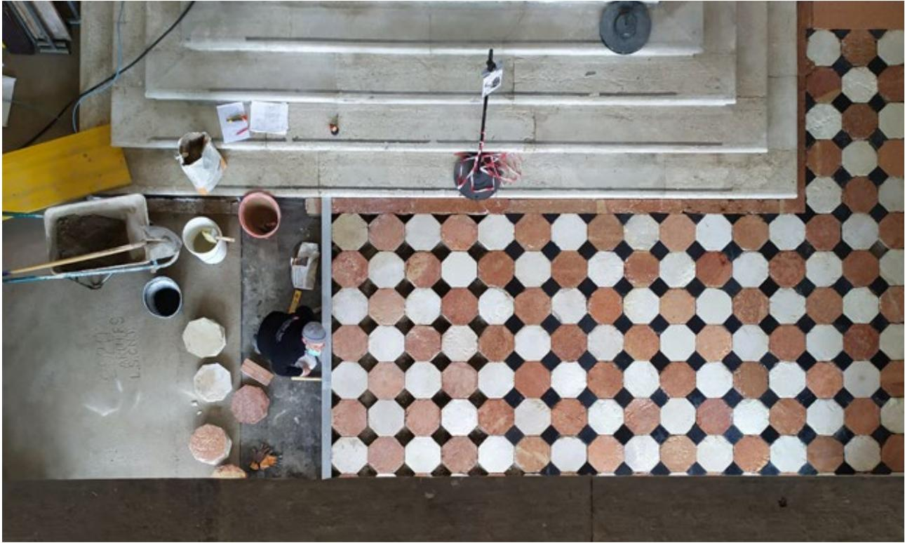
FIG. 3 Dismantling and repositioning the floor octagons
