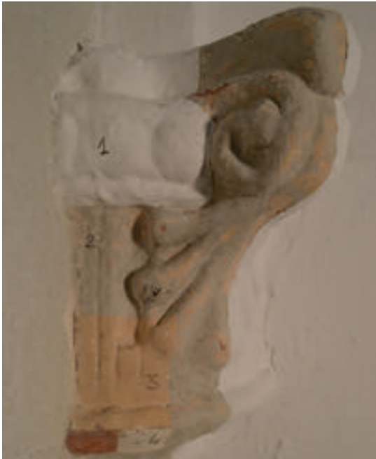
Stratigraphy of a corbel in a side cell highlighting the period whitewashing and the various layers overlapping the original one
