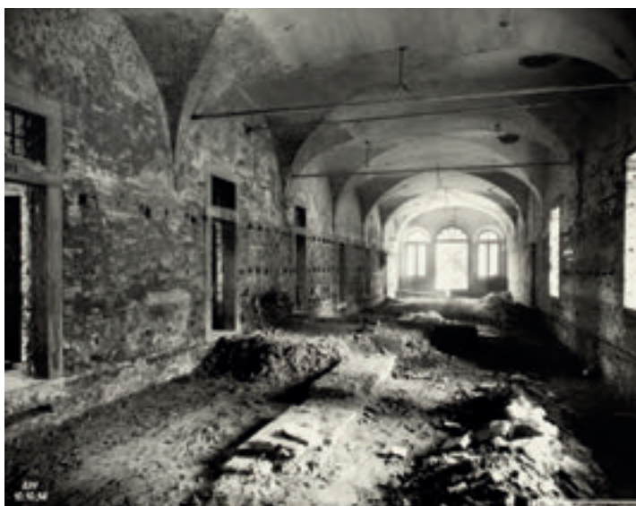
The Messina Room in 1952 during the restoration work. Note the doors equipped with fanlights, the absence of windows, the central opening on the short side still present, the lowered floor and the door that led to the cloister, no longer visible today
