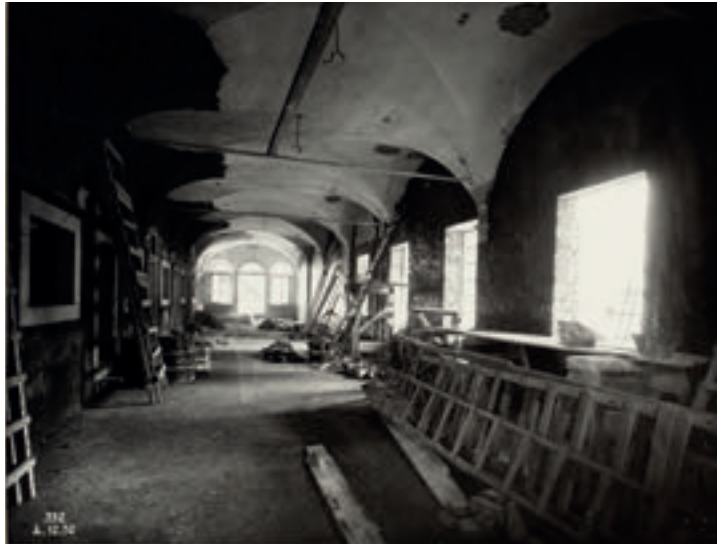
The Messina Room in December 1952 during the restoration work. The window openings have Istrian stone frames and the layer of tar reaches up the walls as far as the vaults
