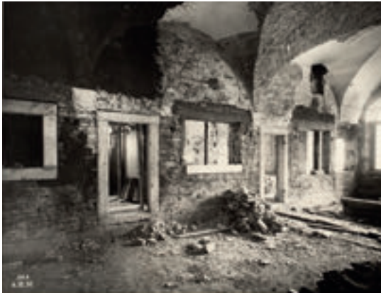
The Messina Room in December 1952 during the restoration work. The window openings have Istrian stone frames and the layer of tar reaches up the walls as far as the vaults
