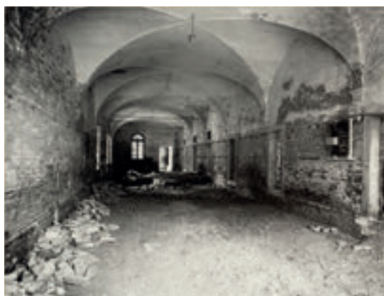
The Messina Room in 1952 during the restoration work. Note the doors equipped with fanlights, the absence of windows, the central opening on the short side still present, the lowered floor and the door that led to the cloister, no longer visible today
